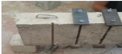
Fig. 5 Install NSM steel bars in the laboratory
