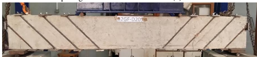
(c) Inclined bars (45°) at 200 mm spacing measuring at bottom of the beam
