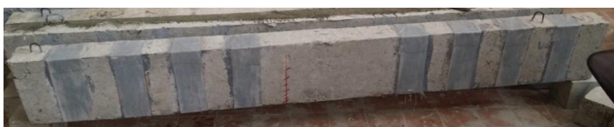
Fig. 9 Strengthening preparation of Beam B2GF-EV20F used externally bonded GFRP strips
